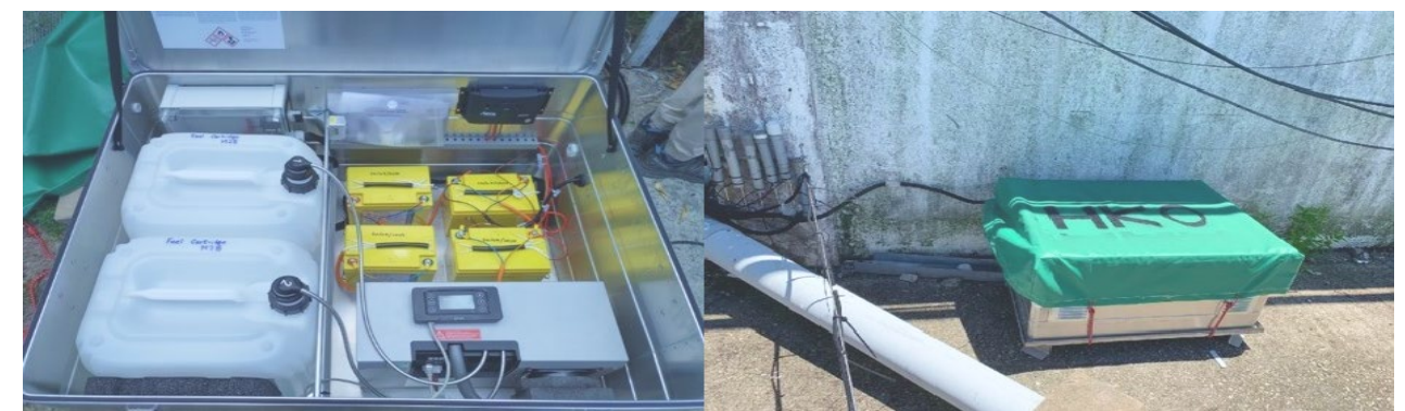
Use of Direct Methanol Fuel Cell at the outstations
