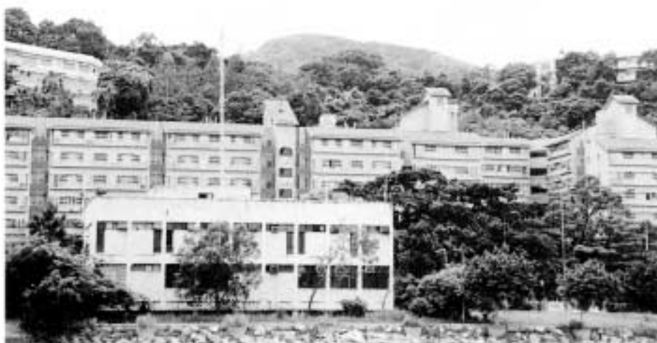
Fig. 3(a). The anemometer mast on the roof of the Marine Police Station looking towards the southwest.
