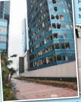
Glass curtain walls were severely damaged on some buildings in Hung Hom.
