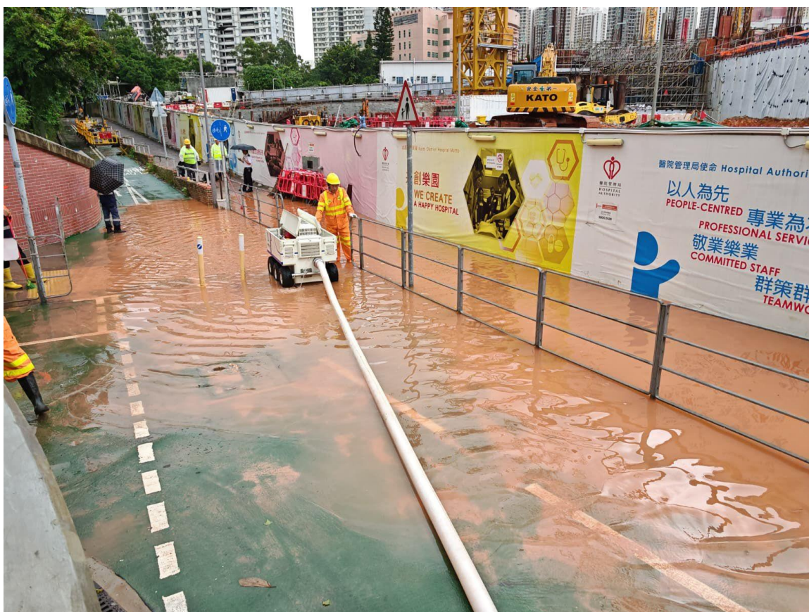
圖 2.2.10 彩園邨/彩蒲苑往粉錦公路行人隧道出現水浸。(鳴謝：渠務署) Figure 2.2.10 The pedestrian subway from Choi Yuen Estate/Choi Po Court to Fan Kam Road was flooded. (Courtesy of Drainage Services Department)
